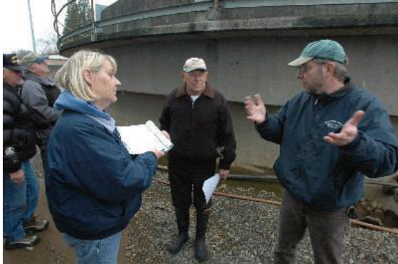
A damage assessment team checks flood damage to the waste water facility in Chehalis, Washington.
